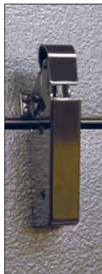
Spring actuated door closer
